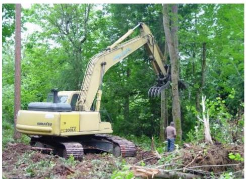
A large excavator parkedout the section of property where I planned to build the garden. Parking-out removed the underbrush and "trash trees", leaving the large Douglas firs without damaging them by rubbing bark off them by pushing logs and brush and stumps around with a bulldozer.
