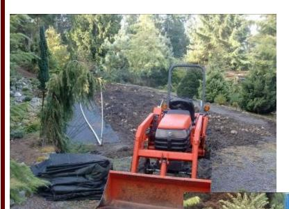
Before building the berms, I subsoiled the garden area. The areas I did not subsoil were reserved for constructing gravel pathways. I laid ground cloth and poured gravel over it. Tha way the gravel would not settle into any mud during the early spring freeze and thaw cycles. I was being extra cautious since I did not have any muddy areas due to the 40% rock content of my soil.
